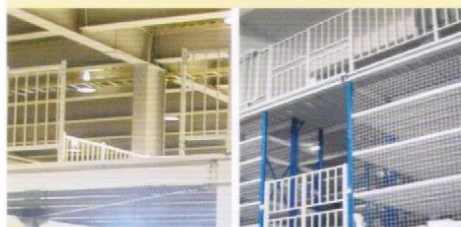
Load and Unload Gate
